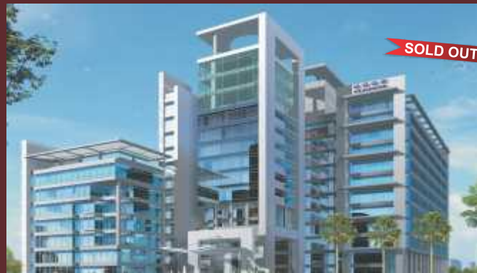
PARK CENTRA, Gurgaon
