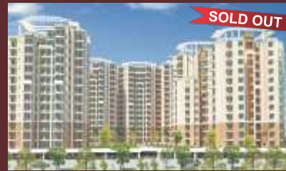
KLJ HEIGHTS, Sector 15, Bahadurgarh
